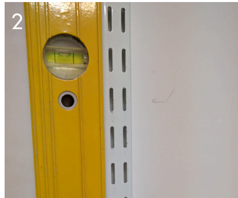
2 Ensure rail is level and continue fixing.
