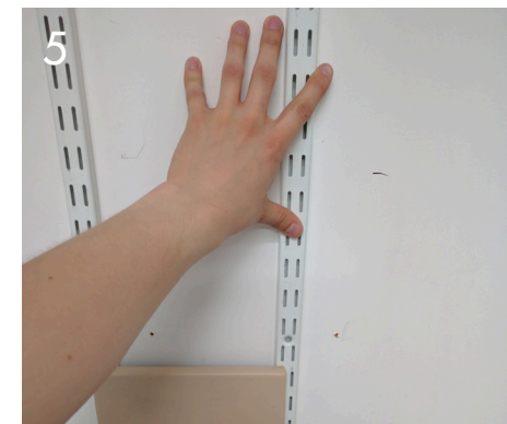
5 Take care that when joining rails vertically, that the distance between the top and bottom slots of new rails are equal to that of all slots on the rails.
