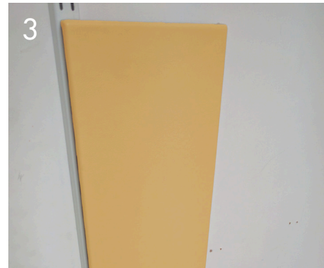
3 Fix next rail into position by carefully using a pitched panel as a guide for distance. Again, ensure rails are level and fix into wall. For the first and last rails, ensure panels slide into the outer slots so that slots are not visible when fully assembled.
