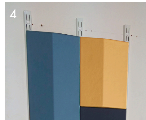
4 Insert panel hooks into rail slots then push down to slide into place. Always ensure that panels are installed starting at the bottom and working up.
